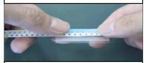
Rub the entire part of the joint tape with your finger to connect tapes completely.
